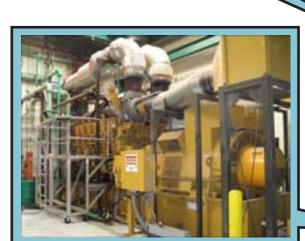
CoGen Facility (Generator) Methane gas is burned to create electricity that runs our plant.
