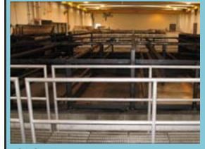
Thickening Sludge is thickened and de-watered before it goes to the digester.
