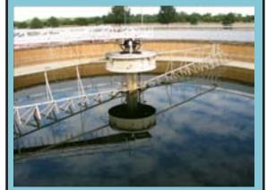
**Primary Clarification Tank** Sludge settles out at the bottom while grease is skimmed off the top.
